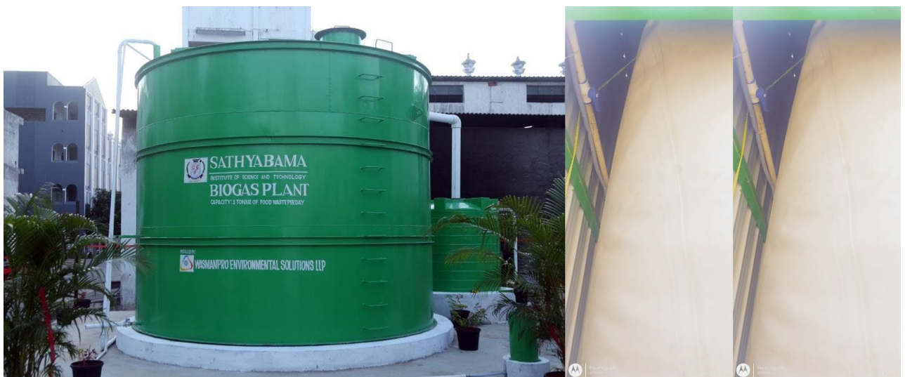
Biogas Plant with 12ft biogas collected in the balloon adjacently diverted for cooking
