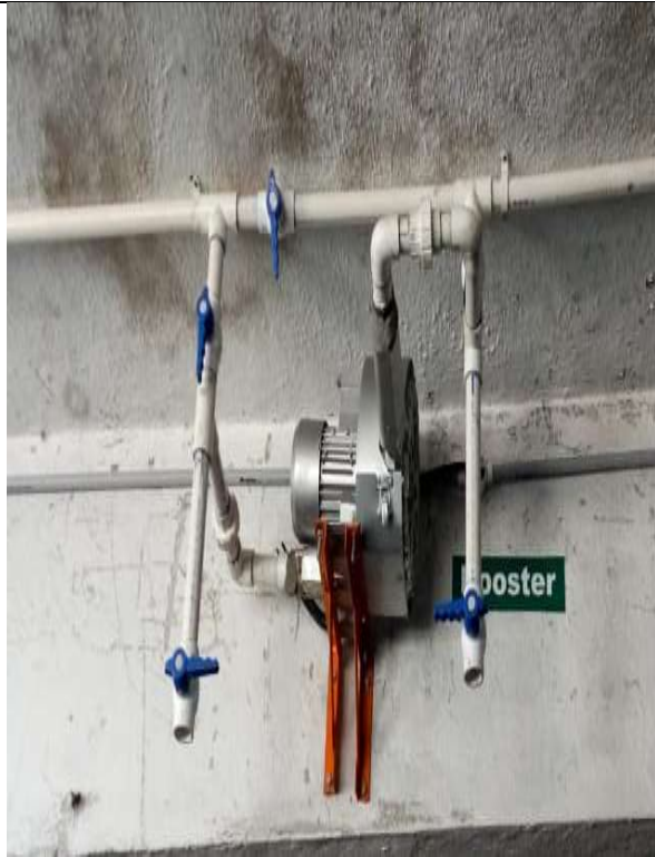
Figure 72: Booster Pump
