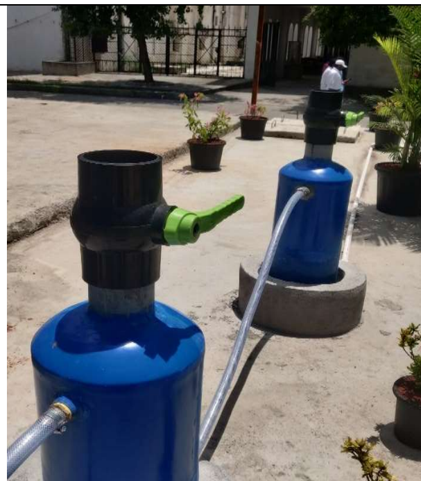
Figure 70: H 2 S Scrubber
