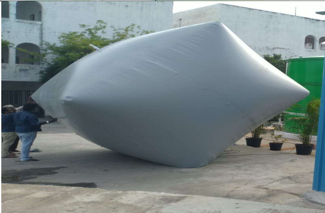
Figure 74: Biogas Storage Balloon
